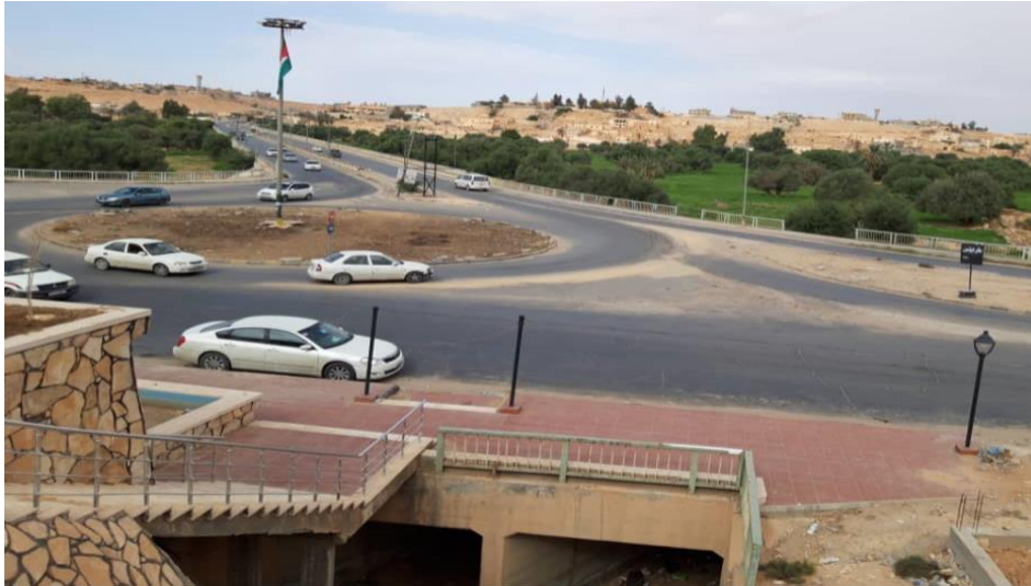
Figure 3: Baniwalid Main Bridge [4].
