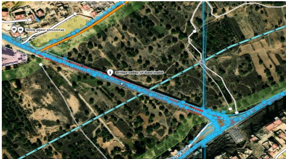
Figure 5: The main bridge.
