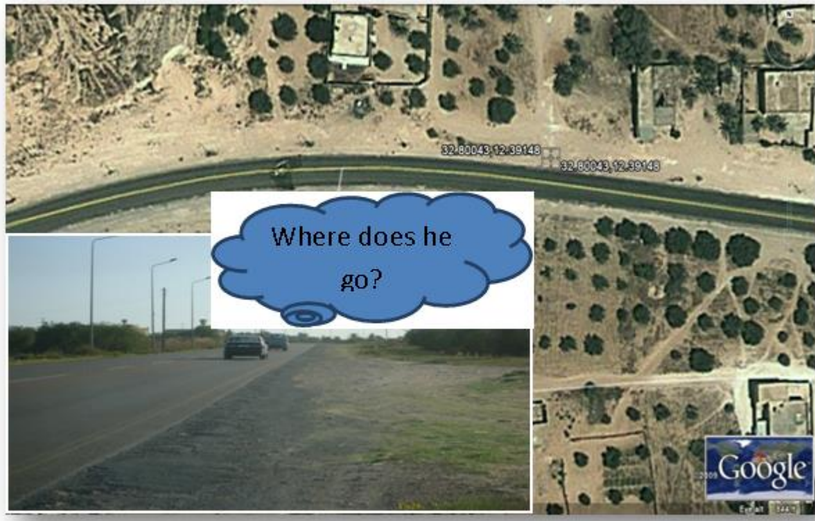
Figure 5. Shown the lack of vision condition of the studied segment
